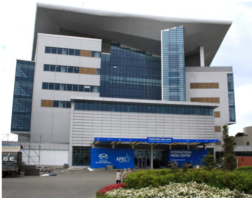
Figure 3. International media centre of Far Eastern Federal University campus.
